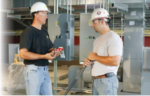
Affected employees Informed power will be off, the reason for it and not to operate equipment
